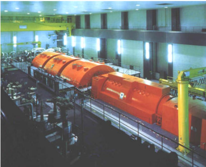
1000 MW Turbogenerator (Siemens/KWU)
